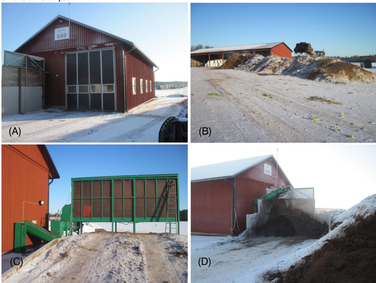
Figure 19. The composting plant at Rölunda farm, which consists of: a) building for the drum composter, b) concrete hard standings for receiving and pre-mixing materials, c) substrate loading container, and d) screw conveyor depositing finished compost.
