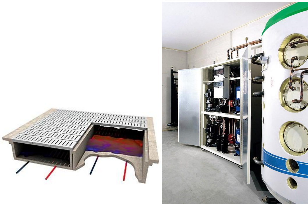
Figure 27. Heat recovery piping is placed in the bottom of slurry channels and connected to a heat pump, which heats water in an accumulator tank ( http://www.pellon.com/In_English/Pig_Husbandry/Heat_pump ).
